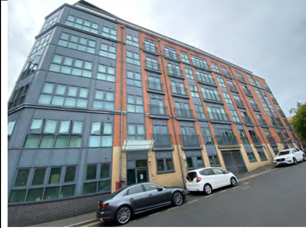
External façade to the front of the property, showing extensive spandrel panels
