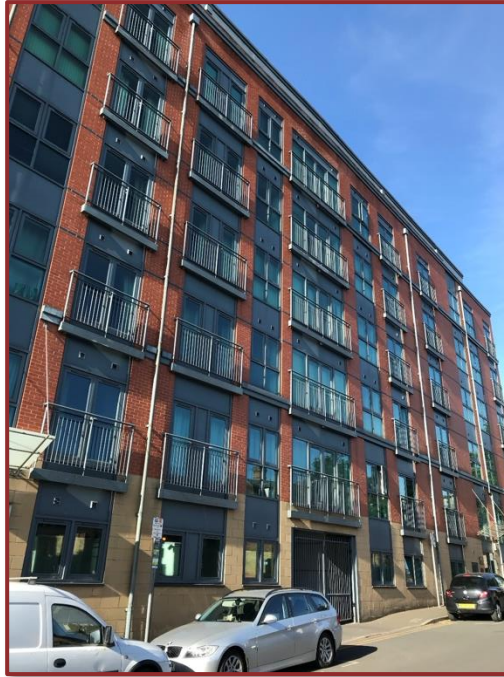
Part North facing elevations to The Habitat consisting of metallic cladding panels, masonry, and balconies.
